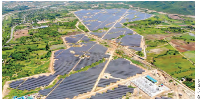
An aerial view of the completed solar farm in Ninh Thuan province.
