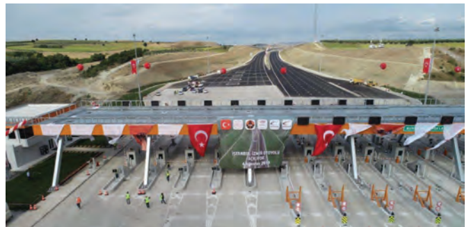
The last section of Gebze-Orhangazi-Izmir motorway is now operational.
