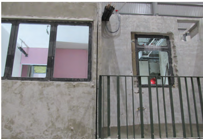
ABOVE, BELOW LEFT AND BELOW RIGHT: PPVC modules for residential projects being stored in Dragages’ new facility at Jurong Port, Singapore. The modules will be completed with internal finishes, fixtures and fittings prior to delivery.
