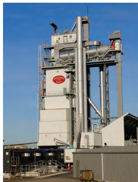
The Ammann ABP HRT asphalt plant incorporates RAP (Recycled Asphalt Pavement) and other recyclable products as the mainstream materials that can produce more than 500,000 t of green asphalt per year.
