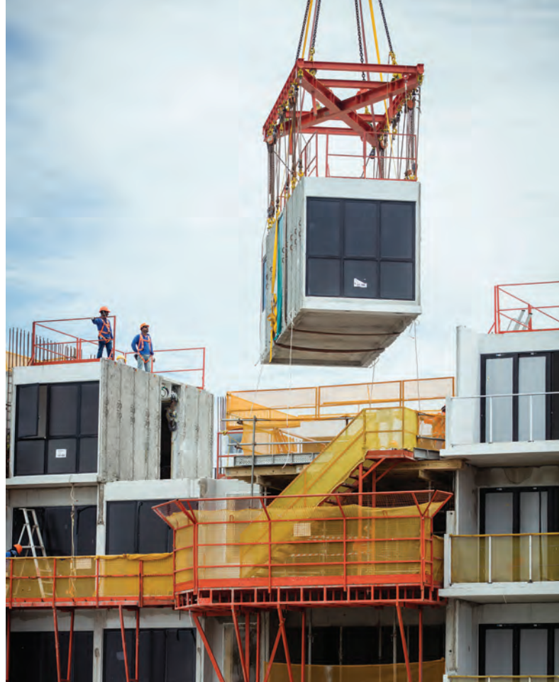
ABOVE, TOP LEFT, LEFT AND BELOW: Lifting and installation of PPVC modules at the Clement Canopy project. These modules had been assembled offsite before they were transported to the jobsite. Dragages adopted the PPVC method for 65% of the building's superstructure.
