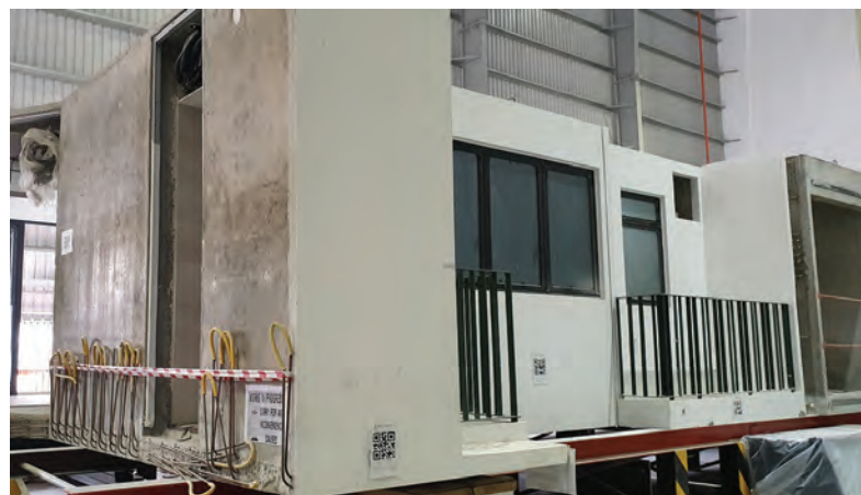
ABOVE, BELOW LEFT AND BELOW RIGHT: PPVC modules for residential projects being stored in Dragages’ new facility at Jurong Port, Singapore. The modules will be completed with internal finishes, fixtures and fittings prior to delivery.
