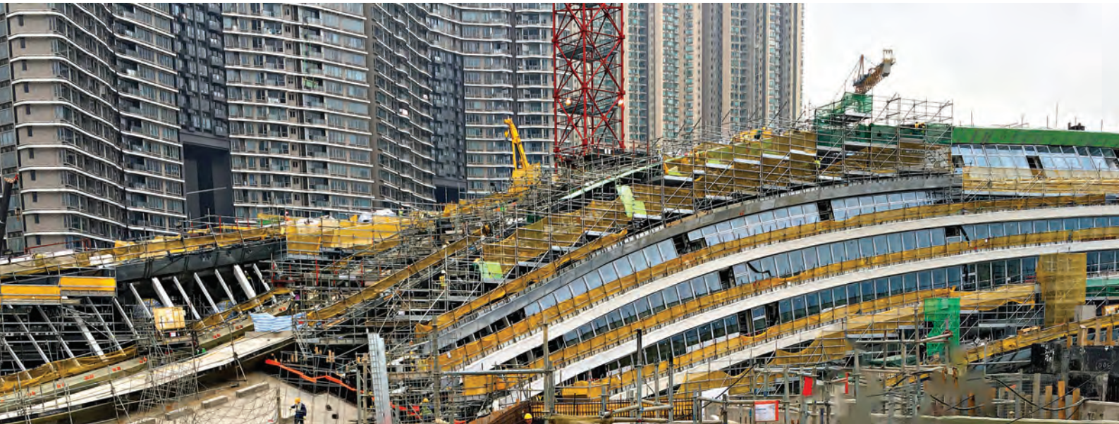
ABOVE AND BELOW: The West Kowloon Station during construction. Aurecon was involved in the planning and managing the erection engineering to raise the long-span station roof to sit protectively and elegantly over 400 000 sq m of rail station.
