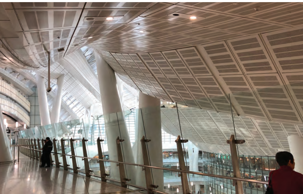
ABOVE: The station's curved steel roof is about 180 m long and 30 m high, supported by six groups of slender load-bearing structures.
