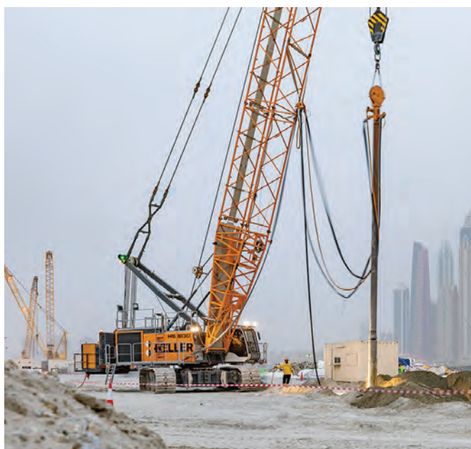
ABOVE AND LEFT: Thanks to the deep compaction work using a Liebherr HS 8130 crane, which is equipped with a vibroflot, Keller is able to improve the building ground down to a depth of 19 m.
