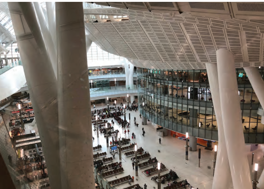
ABOVE AND OPPOSITE: Below the station's curved roof structure is a four-storey building, and above it is a green plaza with nearly 8,900 sq m of open space, accessible by the public.
