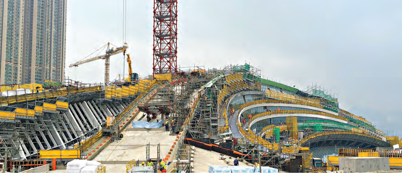
ABOVE AND BELOW: The West Kowloon Station during construction. Aurecon was involved in the planning and managing the erection engineering to raise the long-span station roof to sit protectively and elegantly over 400 000 sq m of rail station.
