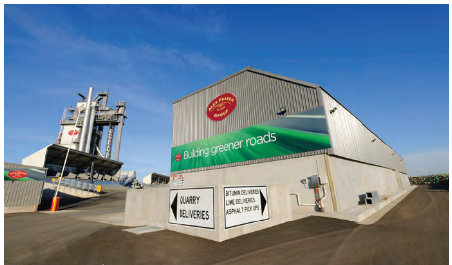
The Ammann ABP HRT asphalt plant incorporates RAP (Recycled Asphalt Pavement) and other recyclable products as the mainstream materials that can produce more than 500,000 t of green asphalt per year.
