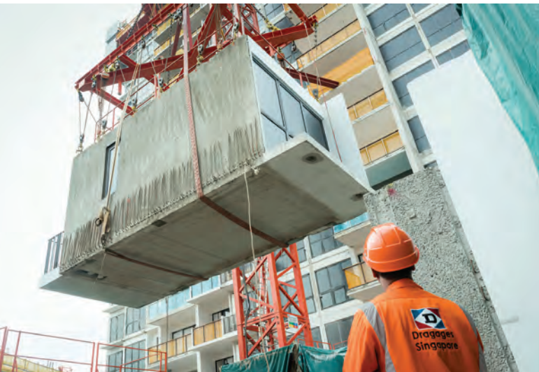
ABOVE, TOP LEFT, LEFT AND BELOW: Lifting and installation of PPVC modules at the Clement Canopy project. These modules had been assembled offsite before they were transported to the jobsite. Dragages adopted the PPVC method for 65% of the building's superstructure.
