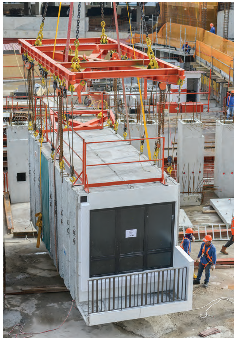
ABOVE, TOP LEFT, LEFT AND BELOW: Lifting and installation of PPVC modules at the Clement Canopy project. These modules had been assembled offsite before they were transported to the jobsite. Dragages adopted the PPVC method for 65% of the building's superstructure.
